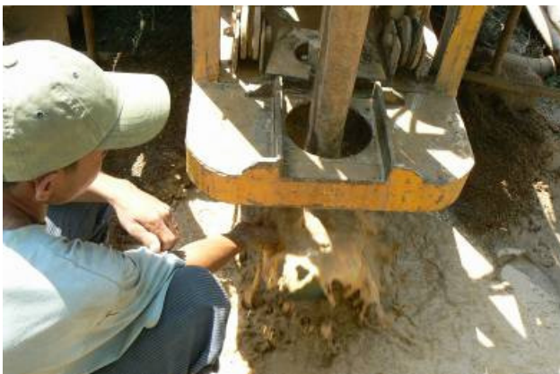
Picture CWPDP: Pump well constructed by Un Somphon Company
